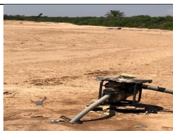
Source: WALP Project
