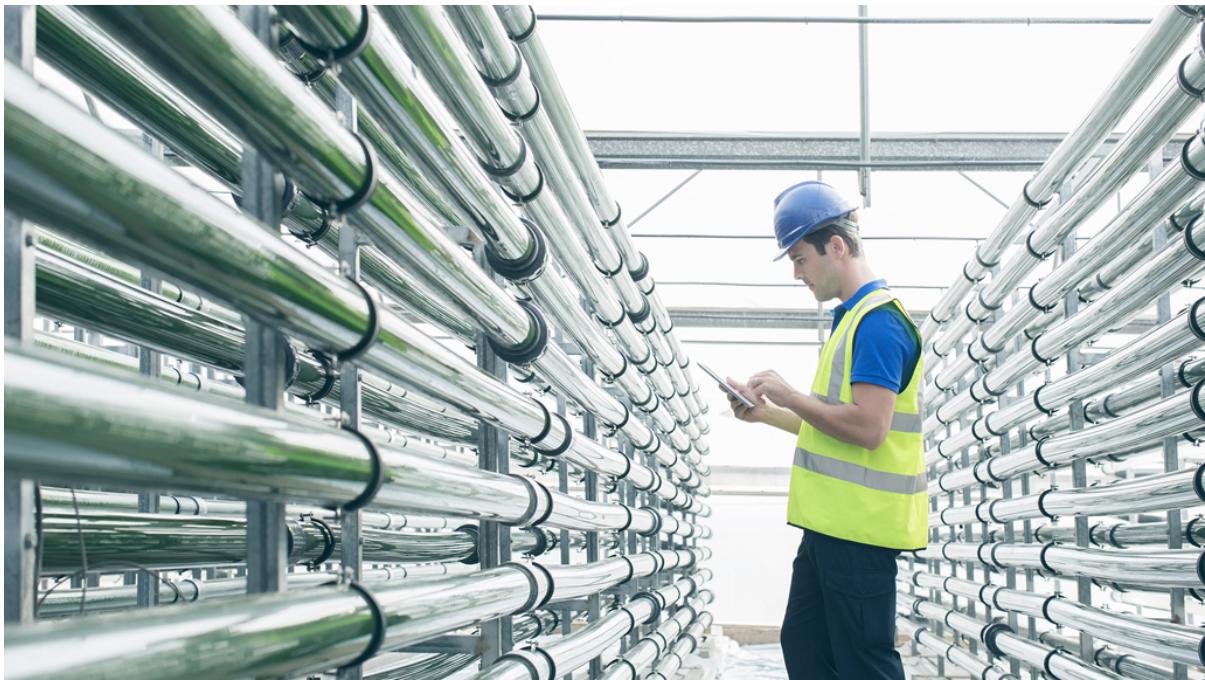
Man with a blue helmet checking a plastic pipe with green algae. | © Caiaimage/Martin Barraud/Getty Images
