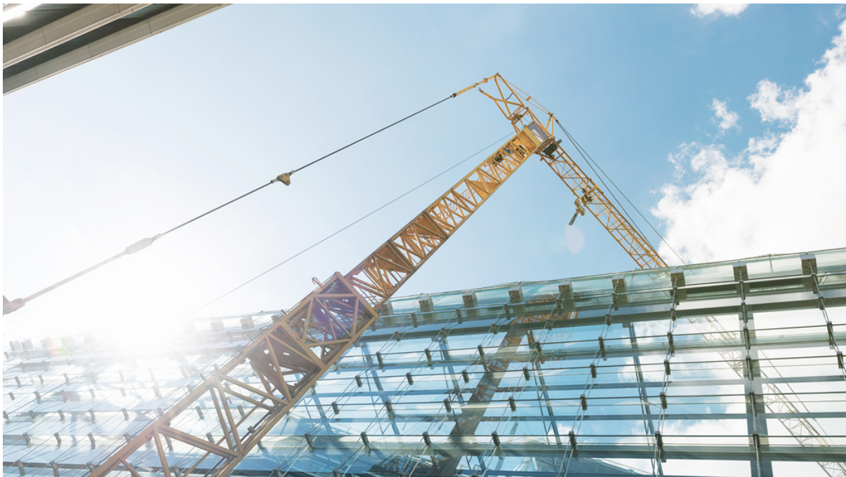
Construction site in Duesseldorf, Germany | © Getty Images/Westend61
