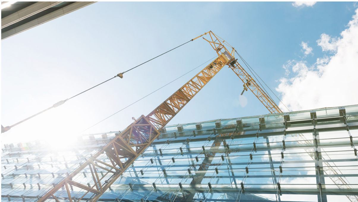
Construction site in Duesseldorf, Germany | © Getty Images/Westend61
